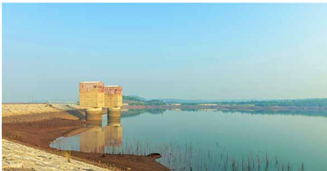
A check dam near Ayodhya Hills, West Bengal
